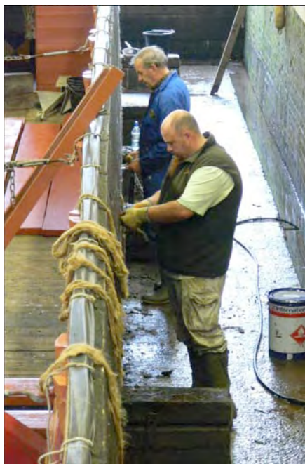
Nick & Neil on the Caulking
