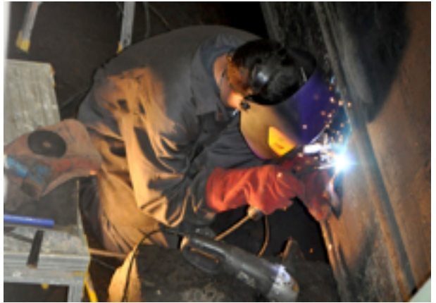
Dale Welding in The New
