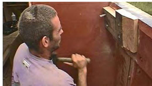
and attaches a beam saddle using the handmade nails.
