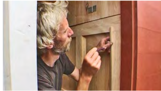
Phil fits beading to the bed cupboard panels.
