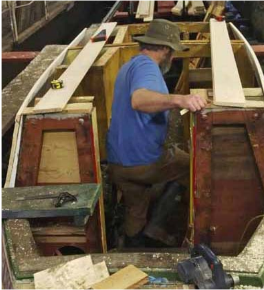
Jem Bates checks the work in progress, 11 Jan 2017
