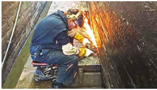
Gavin Clewer cuts back the chine shoe plating
