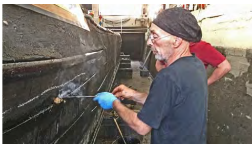
Ade plugs a hole with oakum and tar...
