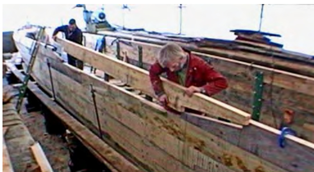
Rebuilding at Tardebigge, February 2000. Picture FoR collection
