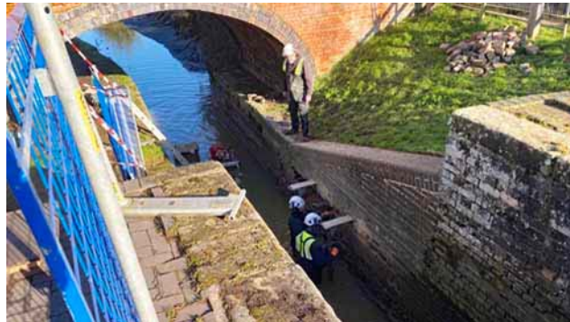
CRT work in progress at Napton Lock 12 on 30th January
