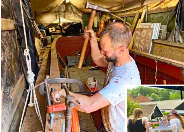
June: new gunwales for Raymond at Brinklow
