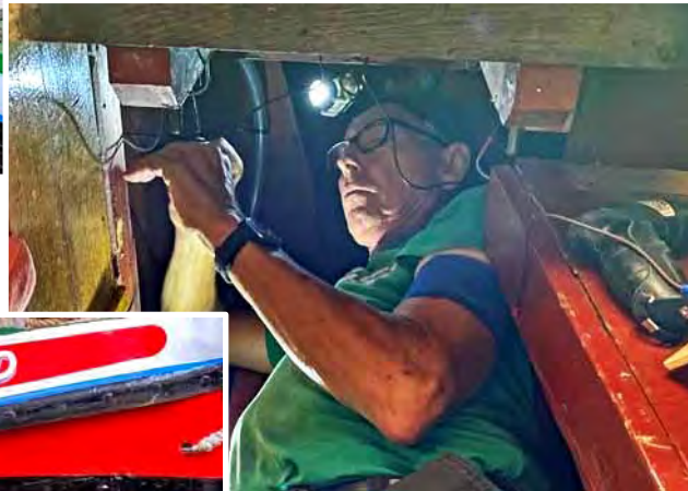
August: Norman fitting stern bilge pumps...
